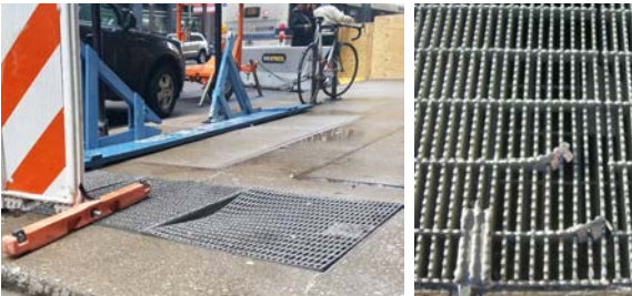
Hazardous Conditions: Damaged Vault Covers
