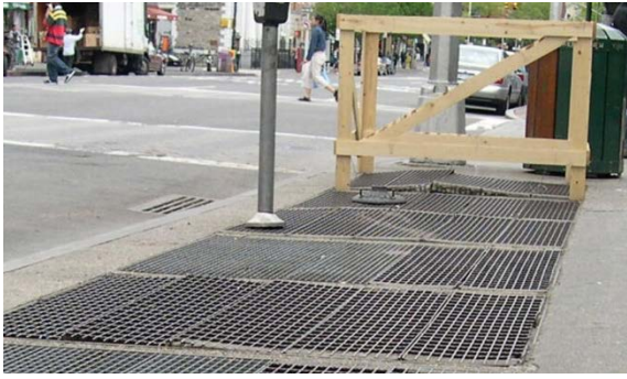
Hazardous Conditions: Damaged Vault Covers
